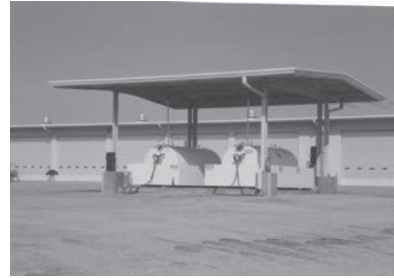
• Fuel island installed at headquarters (above-ground storage tanks)
